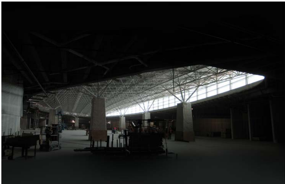
Miami Intermodal Center Construction: Progress Photo February 13, 2009 Rental Car Center (RCC): FM # 249937-5 Construction of RCC Lobby
