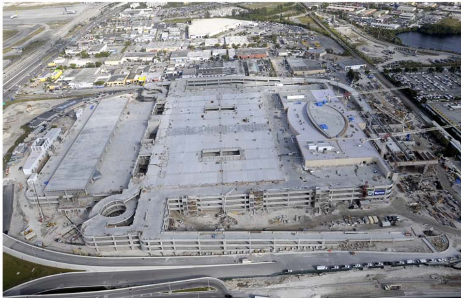
Miami Intermodal Center Construction: Progress Photo January 27, 2009 Rental Car Center (RCC): FM # 249937-5 Northwest View of RCC Construction Site
