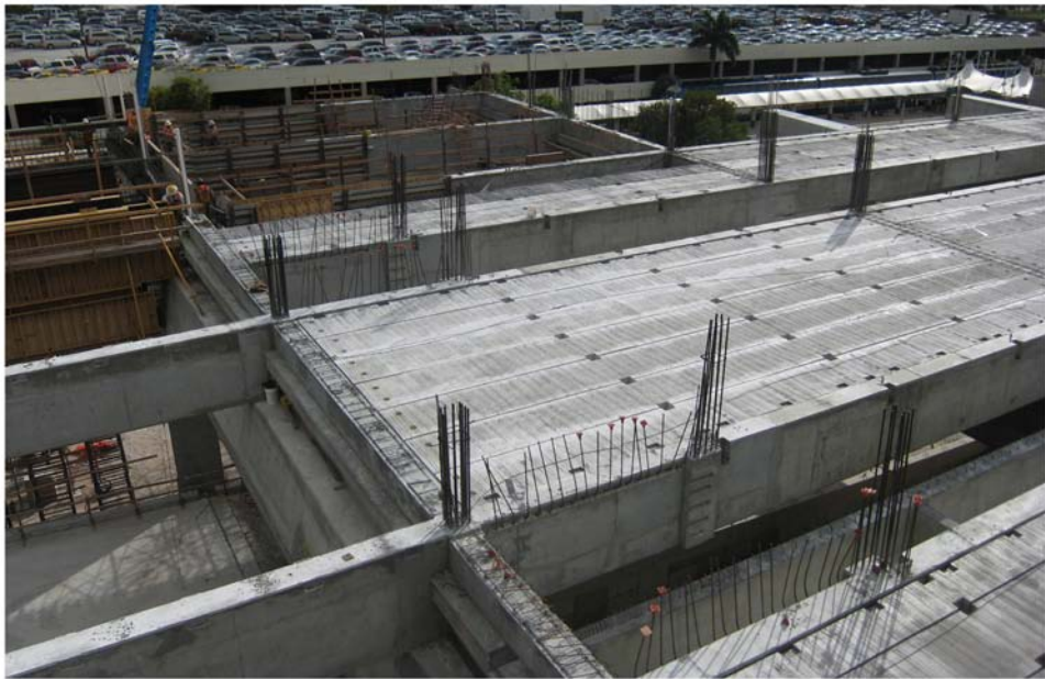
Miami Intermodal Center Construction: Progress Photo January 27, 2009 Rental Car Center (RCC): FM # 249937-5 / MIC-MIA Station: FM # 406800-6 View of MIC-MIA Connector Station Platform Construction
