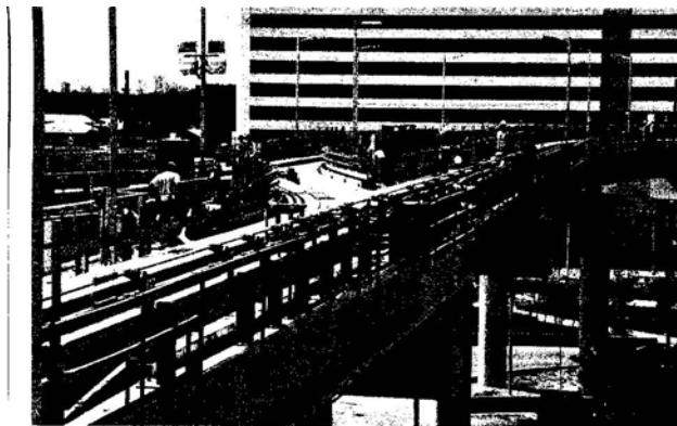
The energized MIA Mover guideway will connect the airport's main terminal with Miami Central Station.
