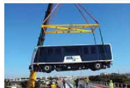
Workers guide the MIA Mover people mover onto the track.
