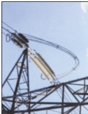
The MIC will work to relocate utility lines for construction
